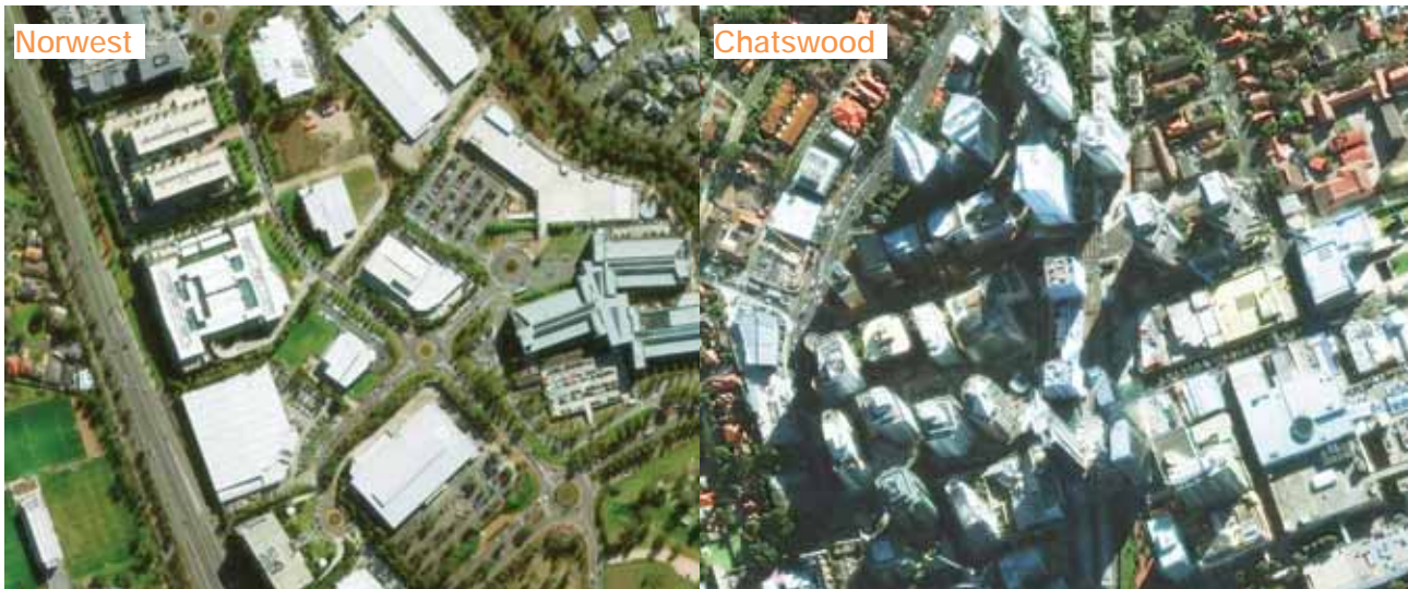
Figure 3 Built form of Norwest (left) and Chatswood (right). Norwest is a car-dominated and car-centric employment centre with a largely inefficient land use allocation. Multiple at-grade car parks are required to serve demands. Chatswood is rail-based centre with higher density employment, residential and retail development. Higher and more productive land uses are located throughout the centre
